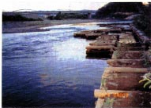
Photo 1 Training works by logs and boulders for improving microhabitat, Toyohira River
